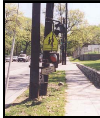
Existing school flasher 28 th Place and 30 th Street
