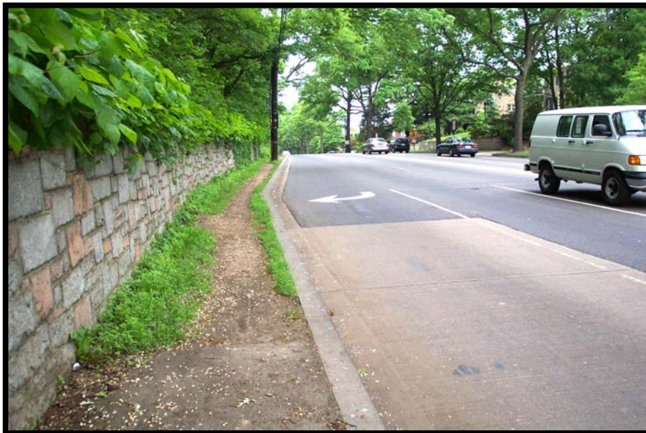
No sidewalk - south side of Pennsylvania Avenue, SE west of Branch Avenue
