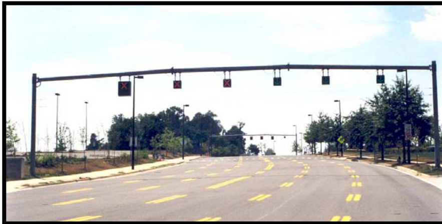
Example of an Overhead Reversible Lane Sign
